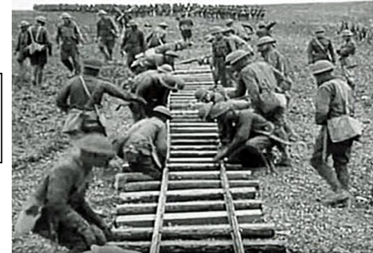
Service Battalion soldiers, or "Pioneers", at work constructing a trench and dug-outs, and laying a line of a light railway.
